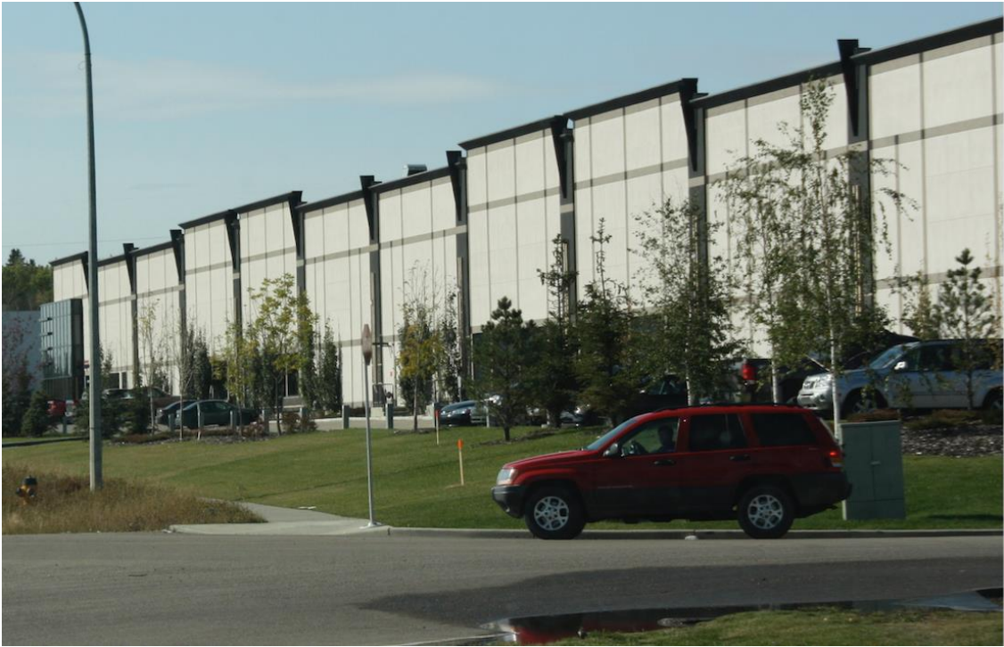
Articulation in the roof line breaks up long horizontal lines
