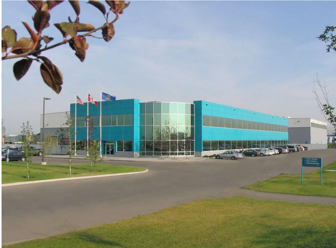
Building massing provides visual interest. Horizontal and vertical articulation and changes in plane occur. Windows have a significant appearance. Focal point indicates building entrance and provides pedestrian scale.
