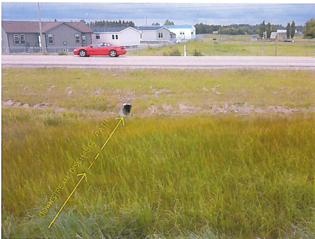
Photo 2: 600mm Culvert under Highway 2A
