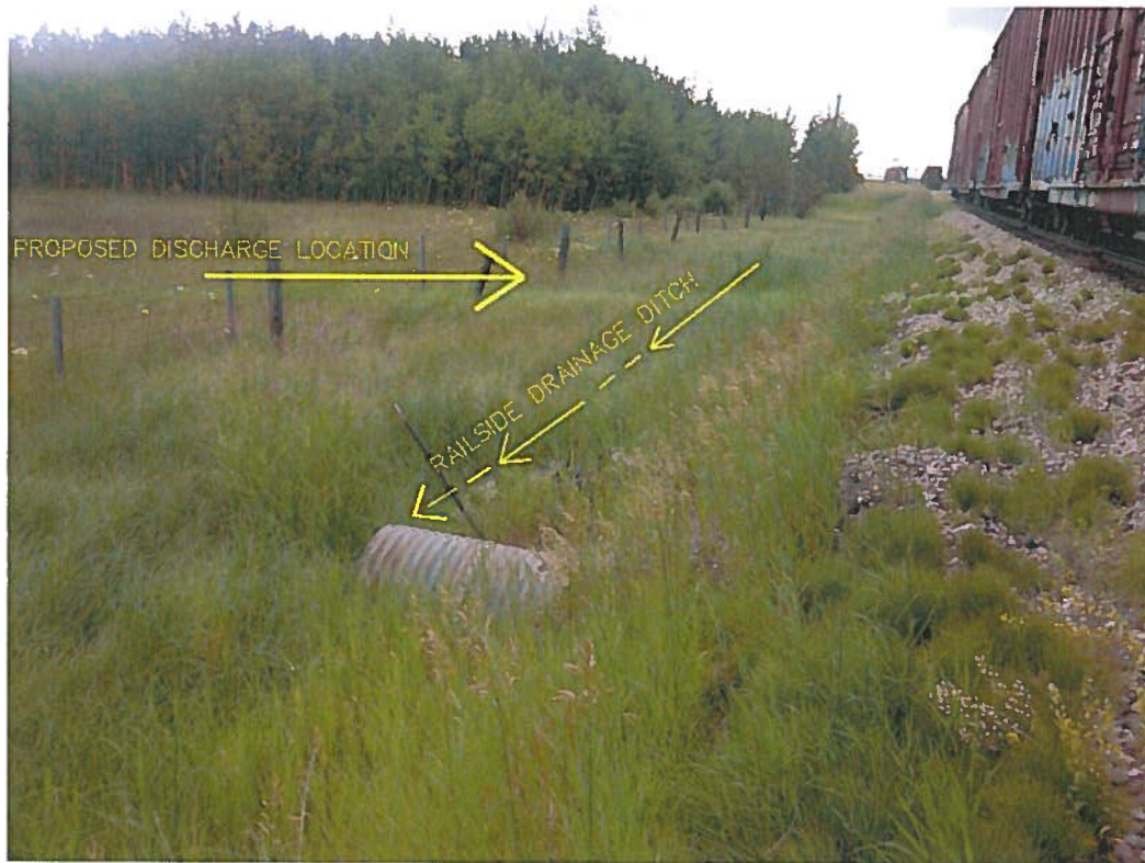
Photo 1: 900mm Culvert under CN Railway
